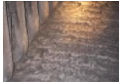
**2. Chunky ash.** Huge "rocks" of agglomerated ash were collected in the Intrex final superheater that required an outage for removal. *Courtesy: JEA*
