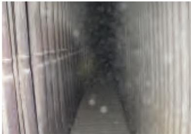
becomes sticky and bonds with other particulate matter that comes in contact with the surface, increasing in size. The process repeats itself to form larger agglomerated ash formations. As the quantity of bonded ash grows, more fuel is required to achieve adequate steam temperatures, reducing the efficiency of the boiler.
